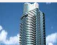
Gargash Tower, Dubai
